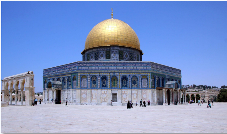
The Dome of the Rock (Qubbat al-Sakhra), Umayyad, stone masonry, wooden roof, decorated with glazed ceramic tile, mosaics, and gilt aluminum and bronze dome, 691-92, with multiple renovations, patron the Caliph Abd al-Malik, Jerusalem (photo: Gary Lee Todd, CC0 1.0)
